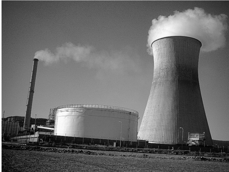
Figure 1: Kühlturm in Form eines Rotationshyperboloids
